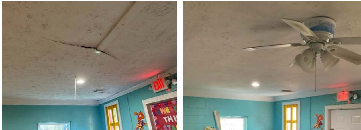
Figure 7. Before and After Ceiling Repair Project
