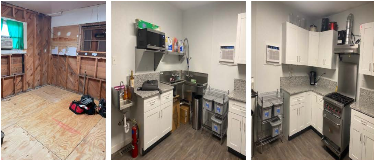
Figure 28. Progress Photos of a Kitchen Renovation
